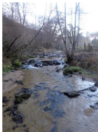
Arasement seuil St Pal
